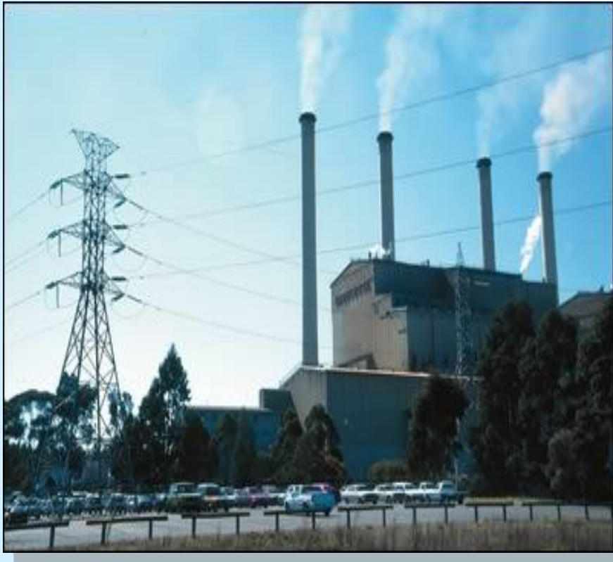
Power Plants Station
